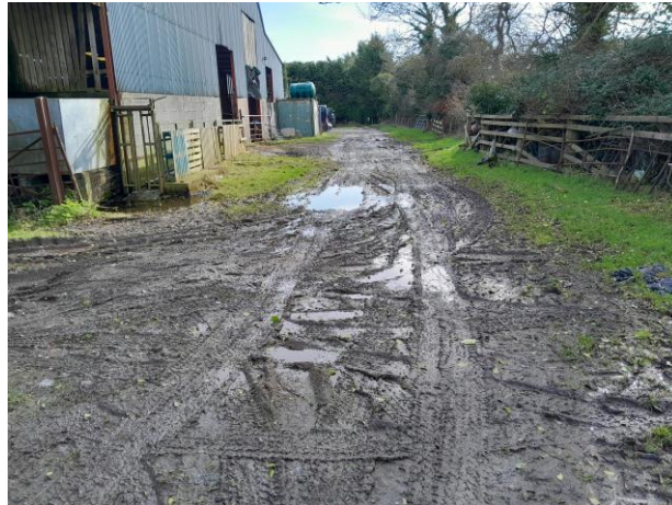
FIGURE 18. EXAMPLE OF ED2 - SPOIL AND BARE GROUND HABITAT AT THE SITE.
